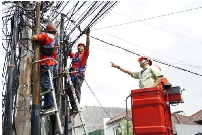
Gambar 1. Instalasi kabel fiber optic
