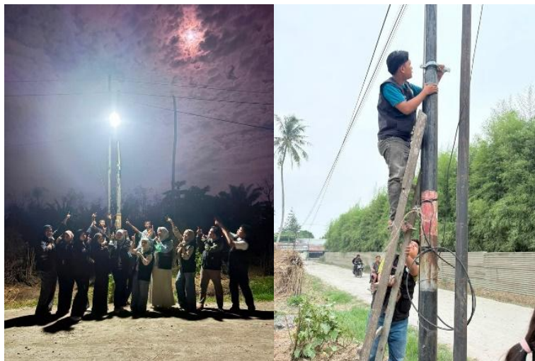
Gambar 1. Proses instalasi lampu tenaga surya
