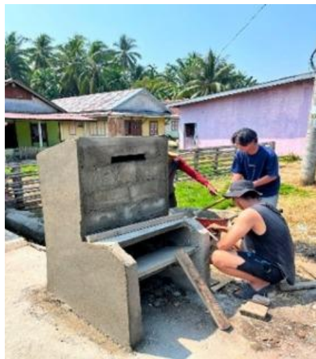
Gambar 3. Proses finishing plester dinding
