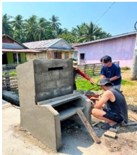
Gambar 3. Proses finishing plester dinding
